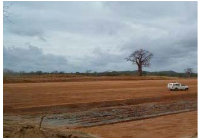
CHPP hardstand final stabilisation in progress
