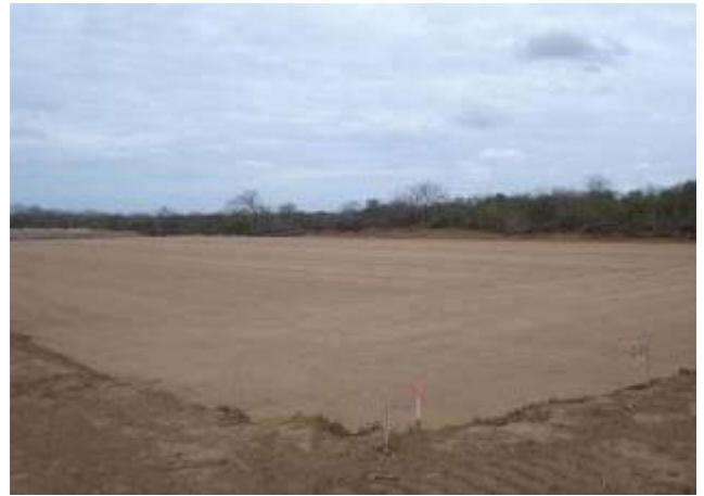
Batchplant terrace ready for occupancy by the Batchplant operator
