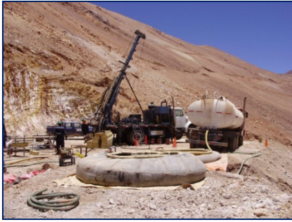
Diamond drilling at Arqueros Sur (geotechnical study)
