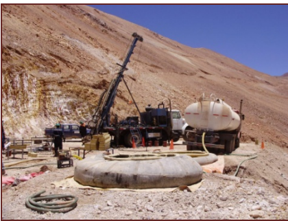
Diamond drilling at Arqueros Sur (geotechnical study)
