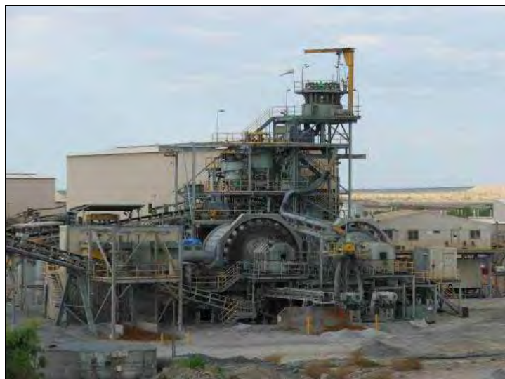
Plate 2. Pillara Plant and associated buildings
