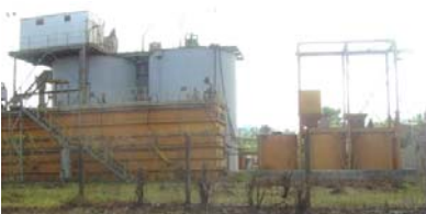
CIL plant located adjacent to Obenemase Deposit
