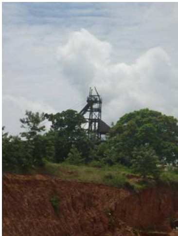
South Shaft, Konongo Mine
