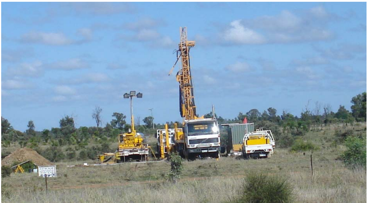
Linc Energy drill rig operation on the Emerald (Teresa) Tenements
